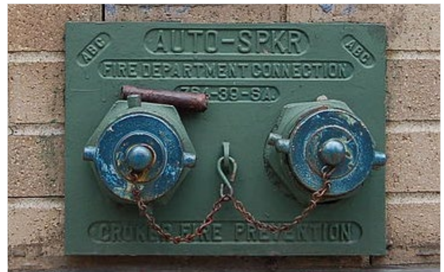
FIGURE 2.1 FIRE DEPARTMENT CONNECTION ON BUILDING
