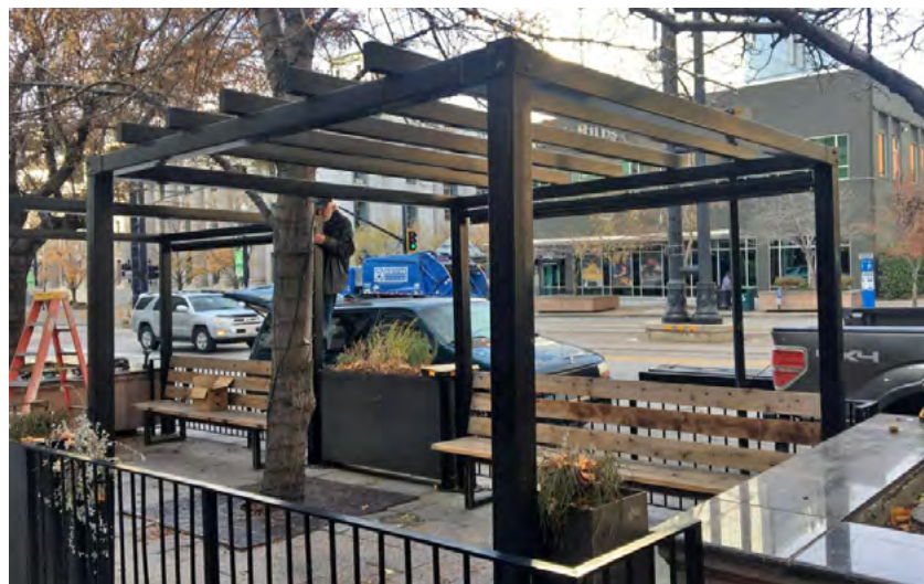
FIGURE 11.3 UNACCEPTABLE COVERING EXAMPLE
