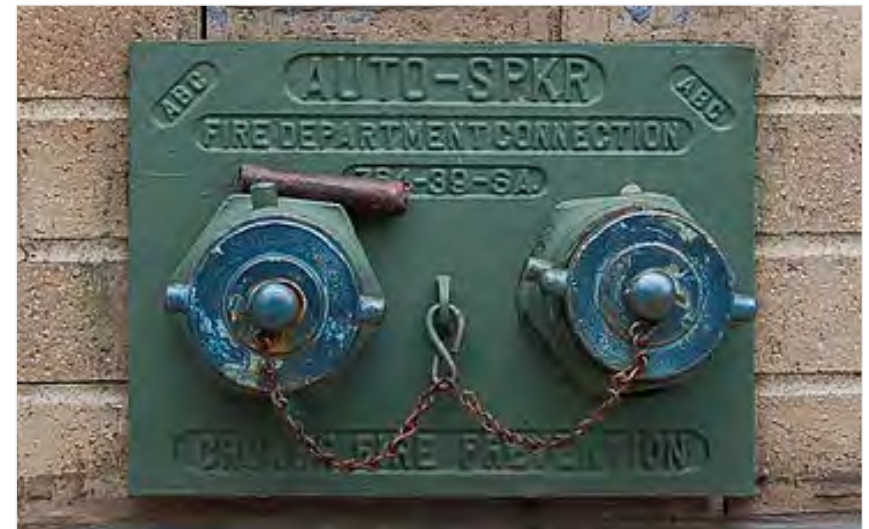
FIGURE 2.1 FIRE DEPARTMENT CONNECTION ON BUILDING
