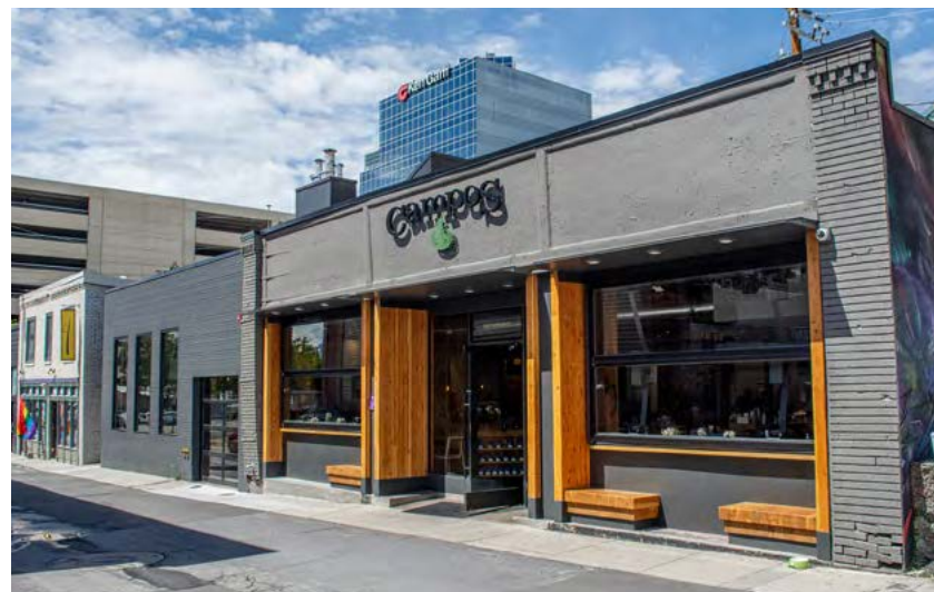
FIGURE 1.11 BIFOLD WINDOWS AND INSET SEATING AT CAMPOS COFFEE, SLC
