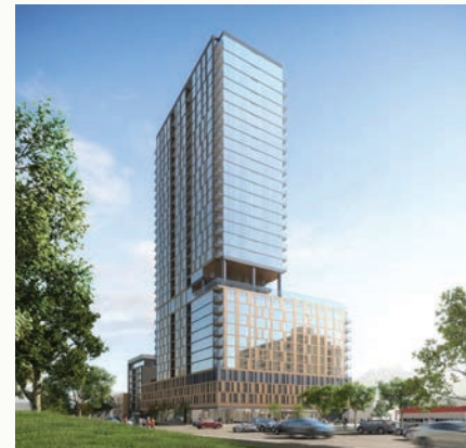
Worthington 200 East 300 South 31 stories, 359 apartments Convexity Properties
