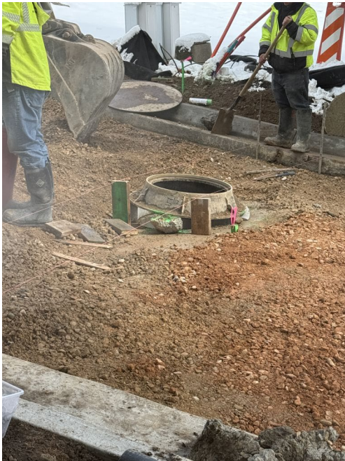
Setting a Manhole on the large PRV Vault
