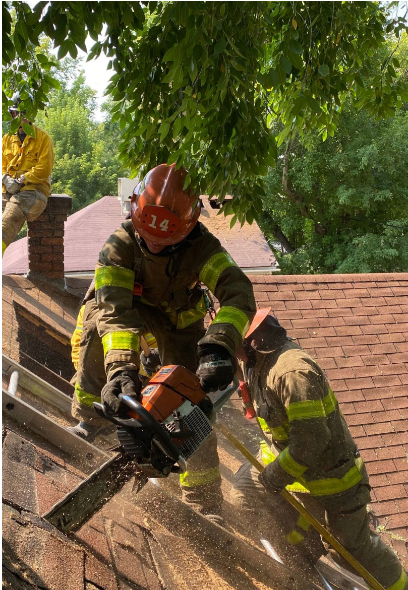
Cutting through a roof with a chain saw.
