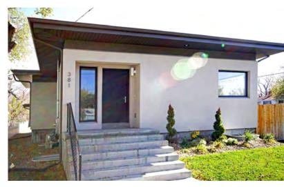
Constructed by HAND, the Emery Passive House is a 2,100 sq ft, 4 bdrm, 2.5 bath home in the Popular Grove Neighborhood. It is Passive House Certified and relies on solar, Energy Star appliances, triple-pane windows, sealed attic space, and insulated basement slab to operate on one-sixth the energy required of a standard home. What's more, it is a HAND Welcome Home Homebuyer Assistance program recipient and placed in the City's Community Land Trust assuring affordability in perpetuity.
