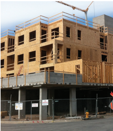
Providing developers who build affordable units a fast-tracked permitting process will decrease the cost of those projects, increasing the likelihood that such projects make it to the market. (Image: VODA)
