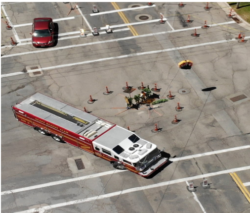
Bottom and right, Pop-up roundabout testing, and completed roundabout. Photo credit SLC Transportation
