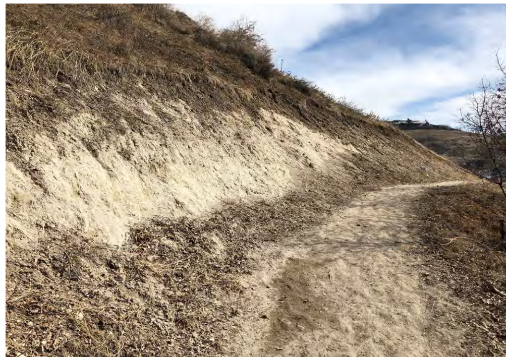
Insufficient specifications for trail design and equipment created unnecessary sloughing and visual impacts.
