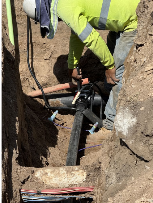
Electrofusing a lateral saddle
