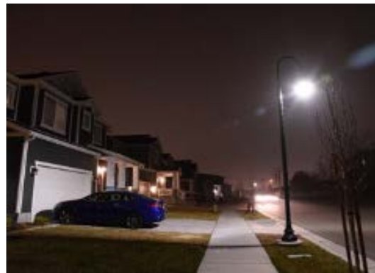
A pedestrian light with inappropriate light distribution and poor shielding creates a significant amount of light trespass on a nearby residence.
