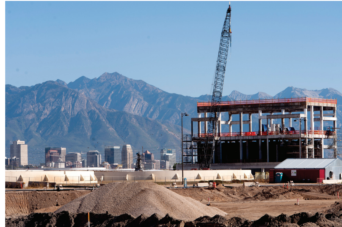
LEFT: Mechanical Dewatering Facility at the new Water Reclamation Facility.
