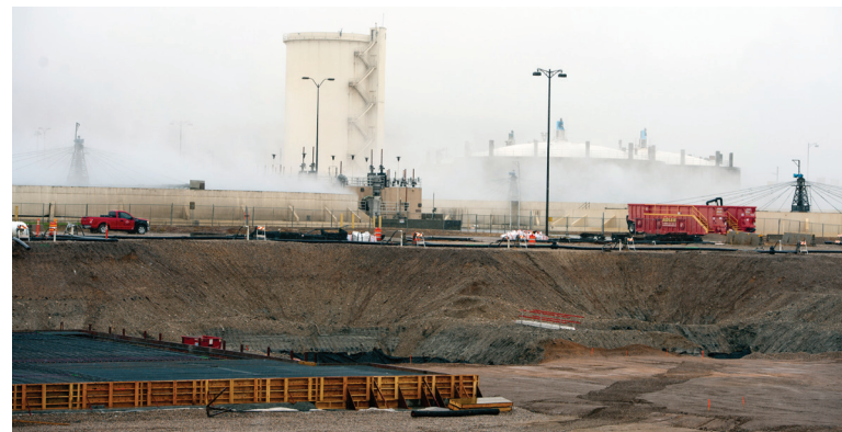
CLOCKWISE FROM TOP LEFT: Mountain Dell construction site. Director Briefer and District Ranger Bekee Hotze work together at a press event in Lamb's Canyon. Crews worked on the Fort Douglas Tank. A foggy morning at the WRF.
