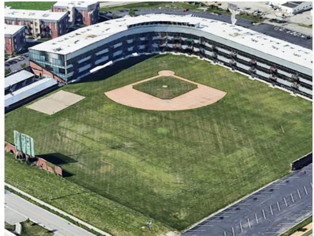
Stadium Village as it looks like today
