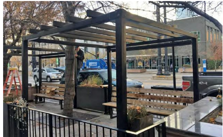
FIGURE 11.3 UNACCEPTABLE COVERING EXAMPLE
