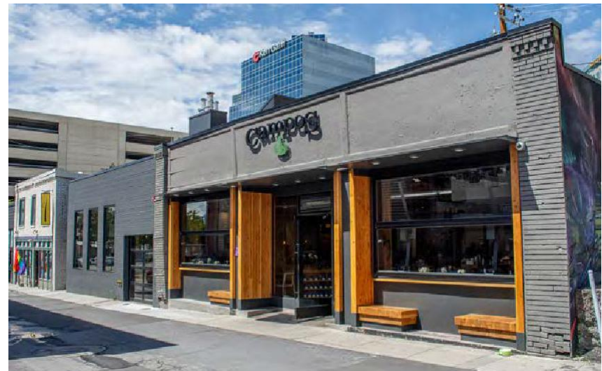
FIGURE 1.11 BIFOLD WINDOWS AND INSET SEATING AT CAMPOS COFFEE, SLC
