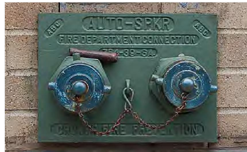
FIGURE 2.1 FIRE DEPARTMENT CONNECTION ON BUILDING
