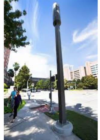
Small cell installations will include attachments on utility poles or lines, traffic signal poles, street light poles, new freestanding poles, or on other structures in the right of way.
