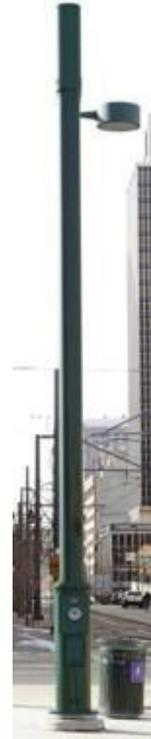
Figure 5-4: Combination Streetlight Pole with Cantenna and Equipment Shroud
