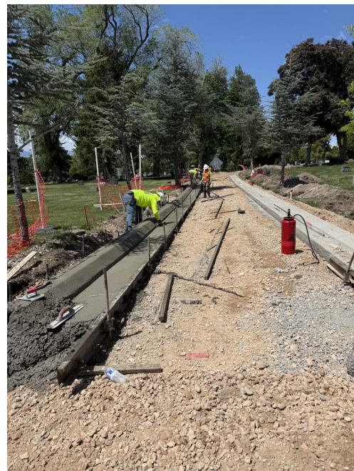
Hand Formed Curb in Phase 8
