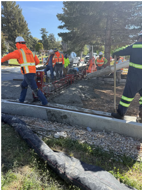
Vibrating Screed in Phase 6
