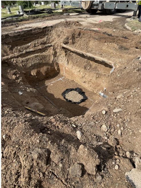
Hole for PRV Vault
