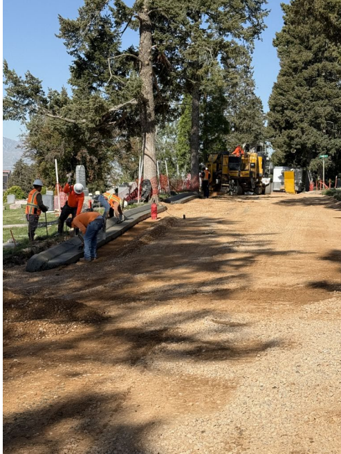
Placing Curb to avoid Tree Damage
