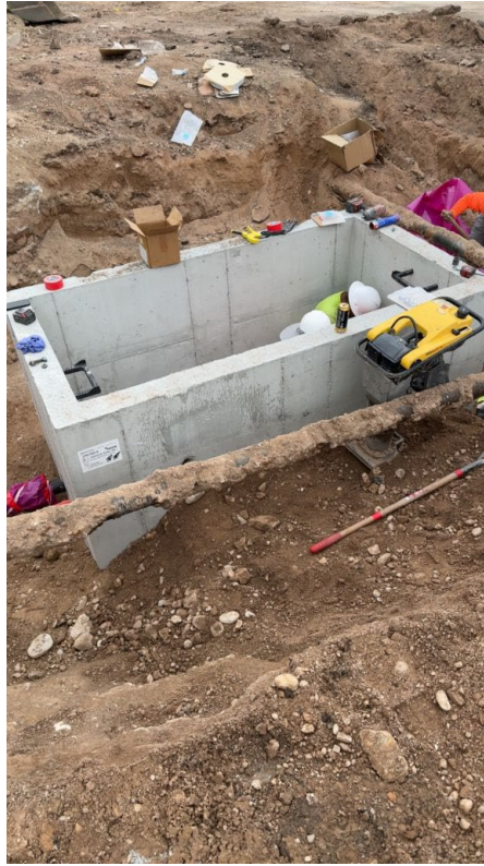
PRV Vault in Phase 9
