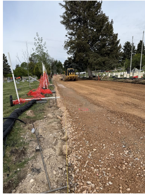
Grading Phase 8, Prepping for Curb
