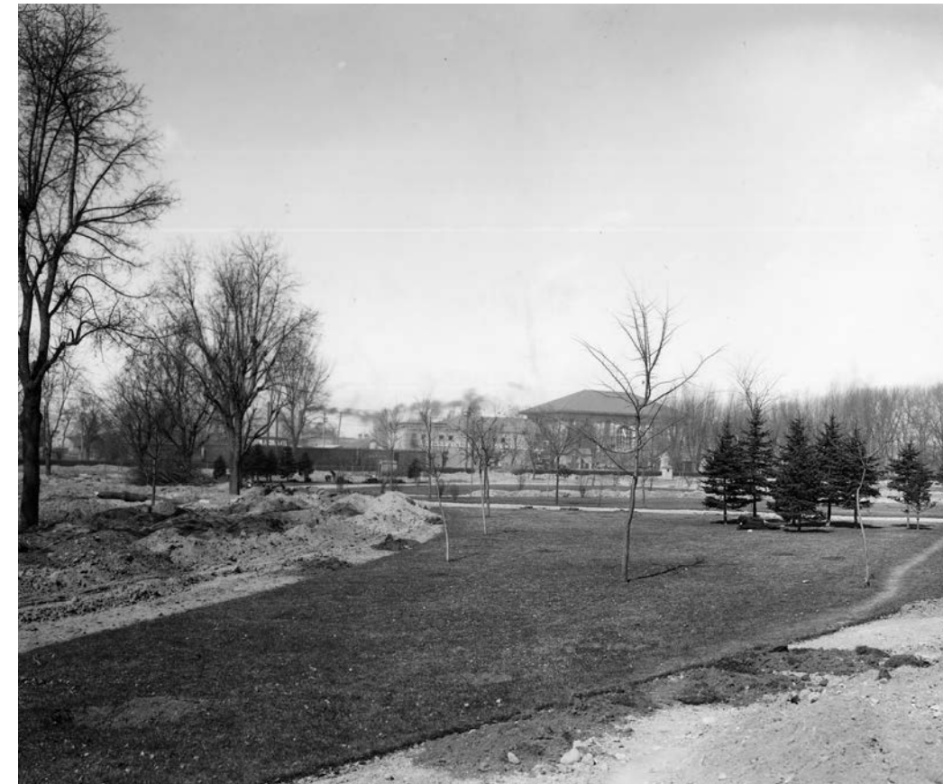
Figure 4-5. Late 1910 photo looking northwest across the park, with the Denver & Rio Grande Depot visible in the background. The piles of dirt visible in the foreground and on the left indicate that this image was taken mid-construction.
