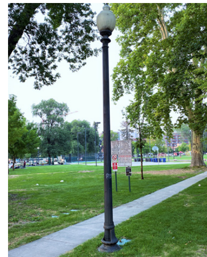
S1. Small light pole
