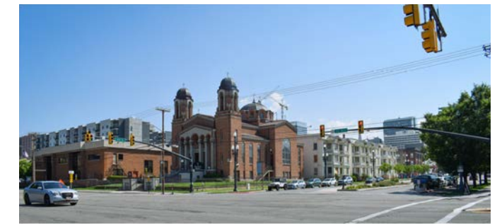
X2. Northeast end, 300 S & 300 W (looking northeast)
