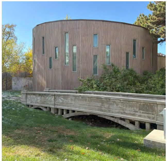
The bridge west of the Concession Building marks the location of a non-extant water feature that conveyed water from Liberty Lake to Swan Pond Tracy Aviary (image: Mundus Bishop, 2025).
