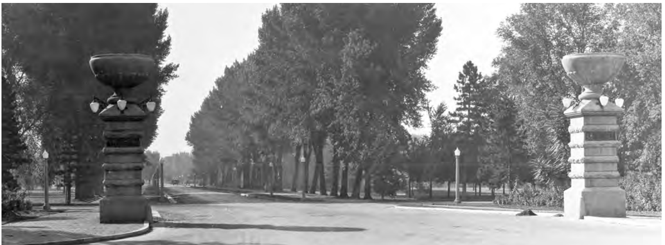
600 E after the addition of monumental entrance piers, lights, curbs, and gutters, before 1918 (image: © Utah State Historical Society).
