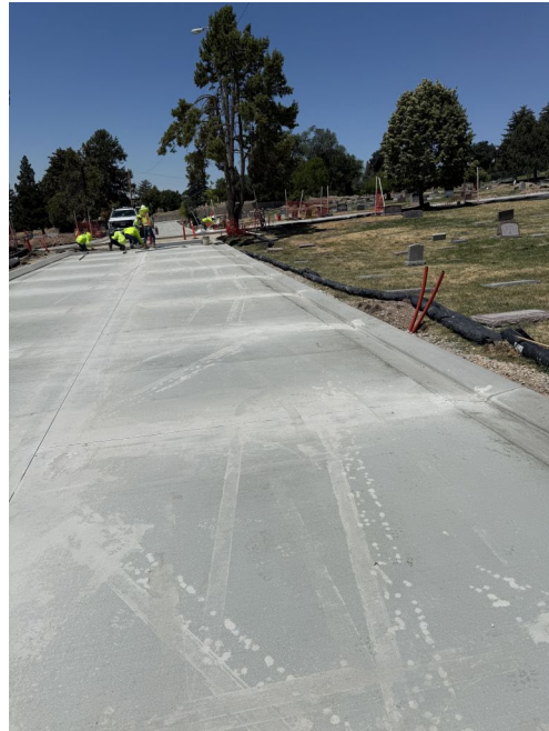
Pavement after cutting, Phase 11
