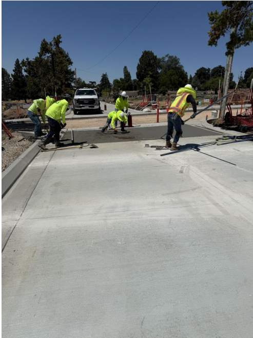
Paving near manholes in Phase 11
