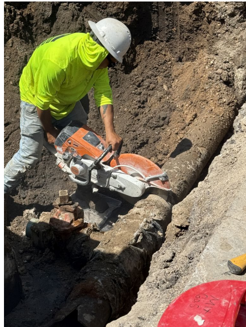
Cutting out the old T junction from the water main
