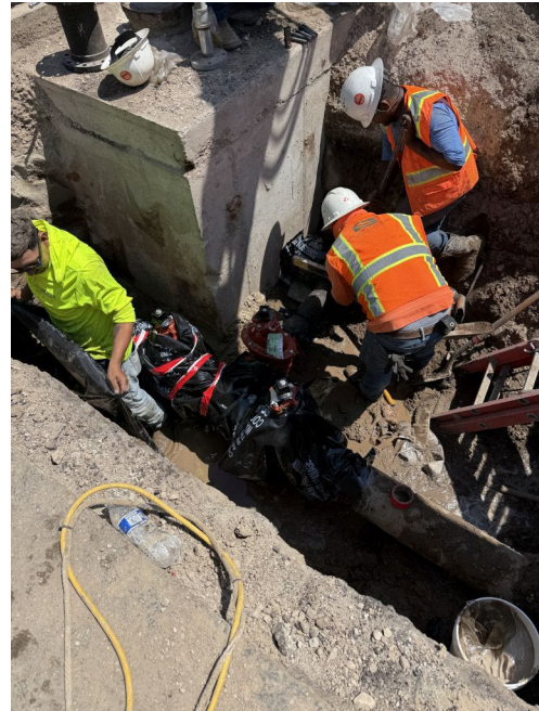
Connecting the water main to the new meter
