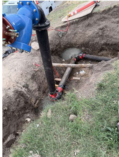
Connecting the water main to the backflow preventer
