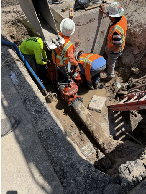
Fitting the new T junction and valves
