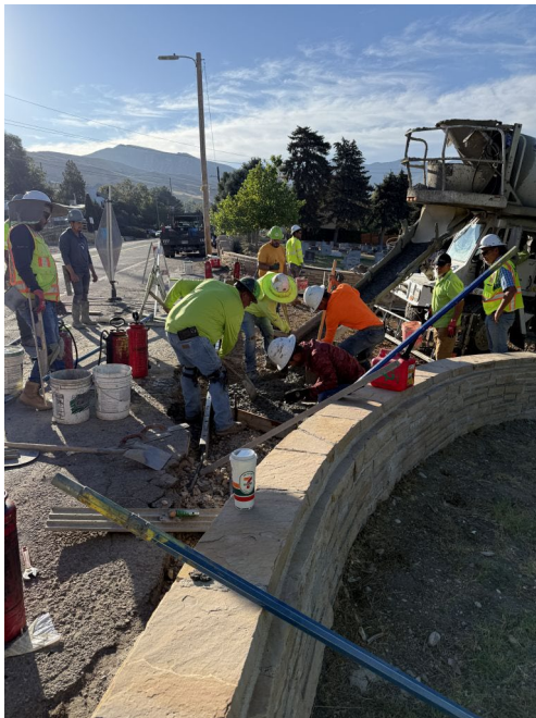
Paving near the East Gate on 11 th Ave.
