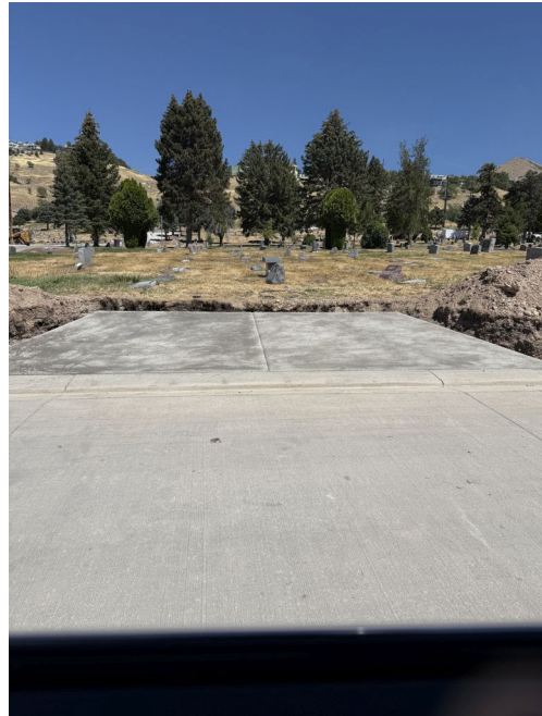
Equipment Access on 325N
