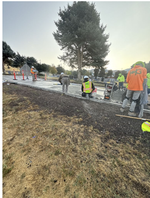
Repouring the same area
