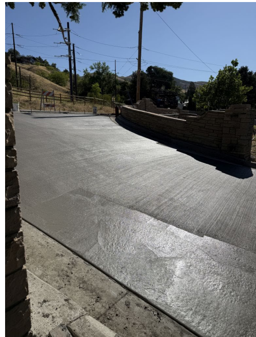
Paving at the East Gate complete
