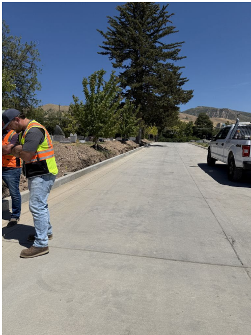
Short wall on 325N due to grade change
