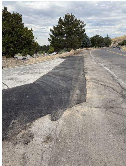
Asphalt tie-in near East Gate on 11 th Ave.
