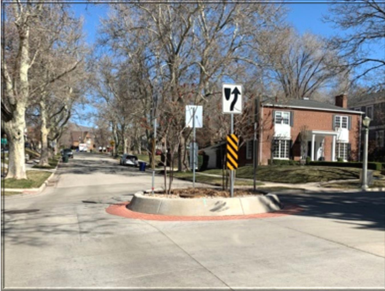
Location: 1700 East & Yalecrest Ave
