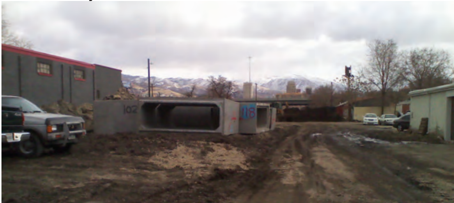
Culvert pipes await installation during the construction of the Folsom Drain Line (Source: Salt Lake City Engineering Department)
