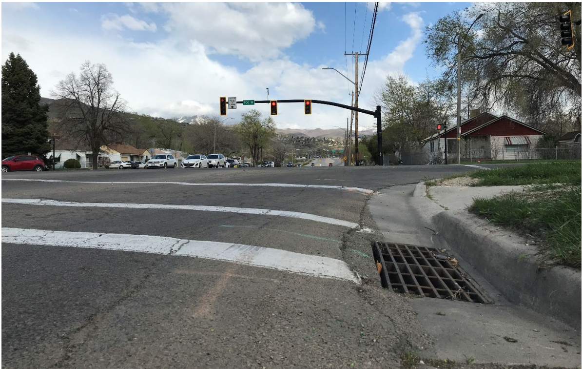
Figure 23: Repeated asphalt overlays combined with steep sidewalk ramps create abrupt dips that make it difficult for pedestrians with wheels to safely cross the street.
