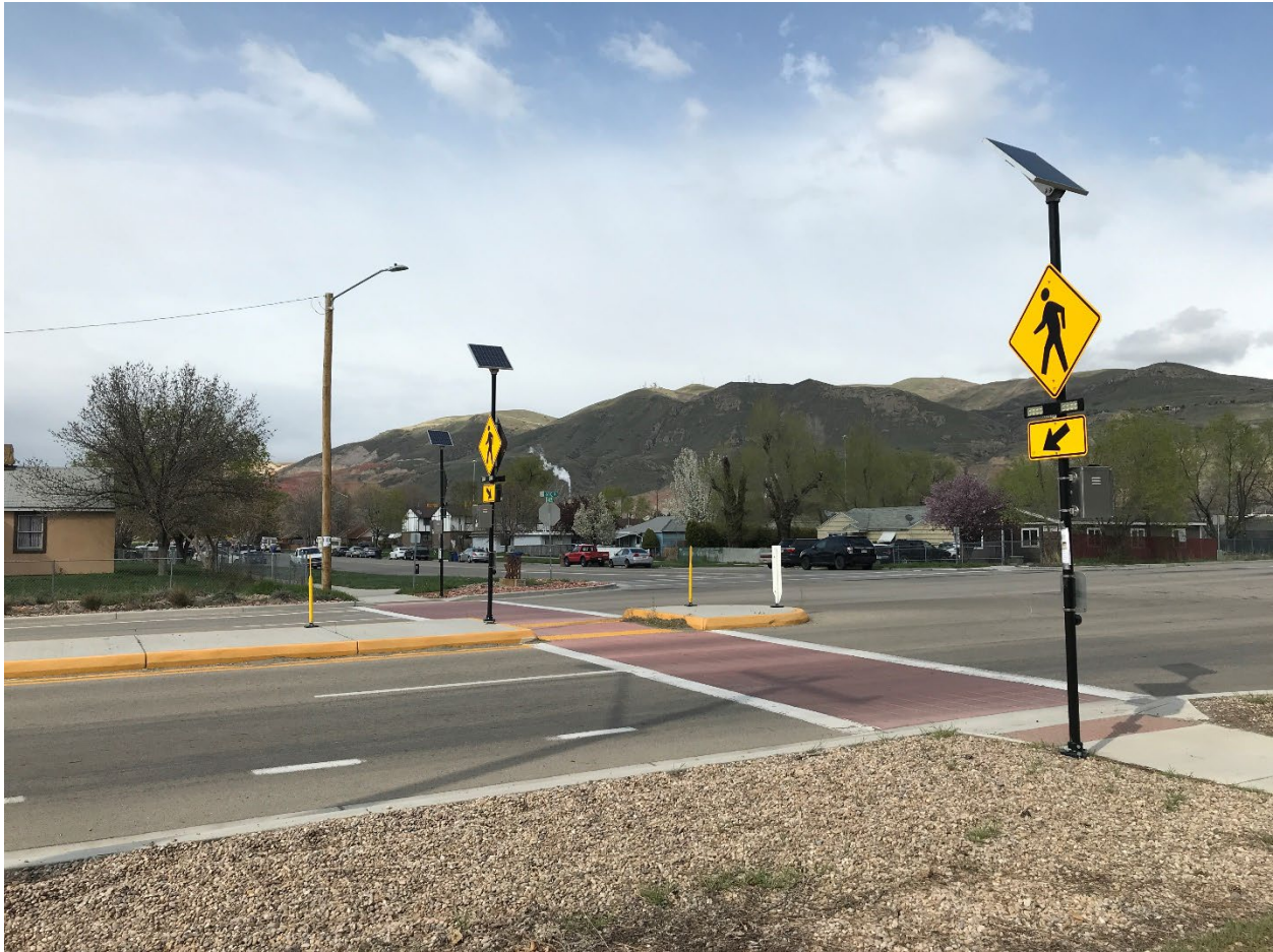
Figure 27: Rectangular Rapid Flashing Beacon at 800 W. Crossing enhancements such as beacons, high-visibility crosswalks, and pedestrian refuge medians greatly improve the comfort of pedestrians and increase motorist yield behavior.
