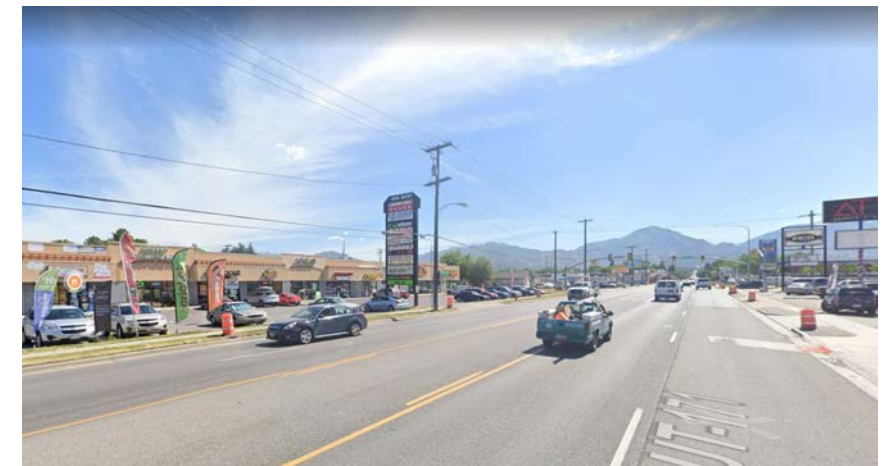
Center Turn Lane and Large Overhead Utilities on North Side
