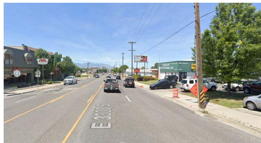
Narrow Sidewalks with No Street Buffer and Utility Poles on Curb
