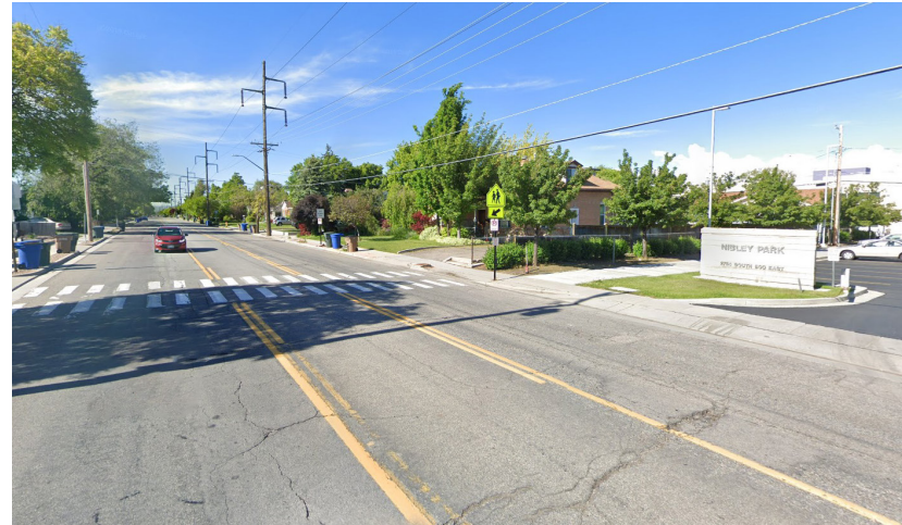
South view of existing 900 East cross section by Nibley Park School.
