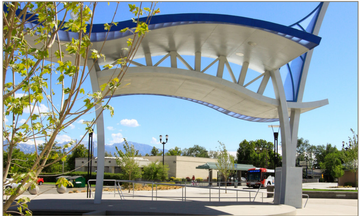
Source: Fairbourne Business Park (top), Wadman Corporation (bottom)
