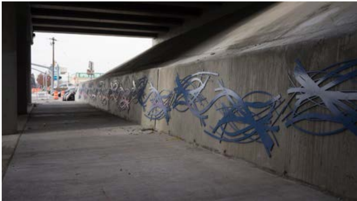
EXISTING SUP ON 1300 S UNDERNEATH I-15, WHICH INCLUDES PLACEMAKING ART
