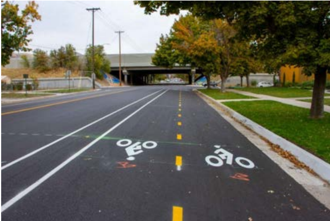
300 N TWO-WAY CYCLE TRACK AS IT GOES UNDER I-15 (SOURCE: SALT LAKE CITY)
