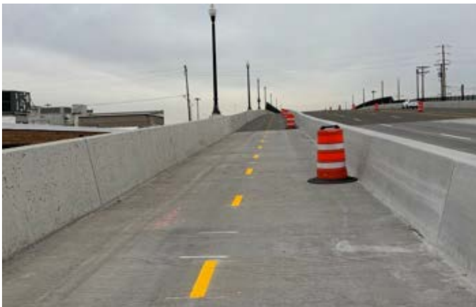
400 S VIADUCT TRAIL UNDER CONSTRUCTION (SOURCE: SALT LAKE CITY)
